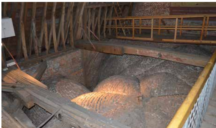
THE UPPER SIDE OF THE GROINED VAULTING OF THE WILLIBRORDUSKERK, DEURNE, SEEN FROM THE CAVITY BELOW THE TIMBER ROOF. THOUGH THIS WAS OF ARCHITECTURAL RATHER THAN MUSICAL INTEREST, IT GIVES A FASCINATING INSIGHT INTO THE TECHNIQUE OF GOTHIC VAULT CONSTRUCTION.
